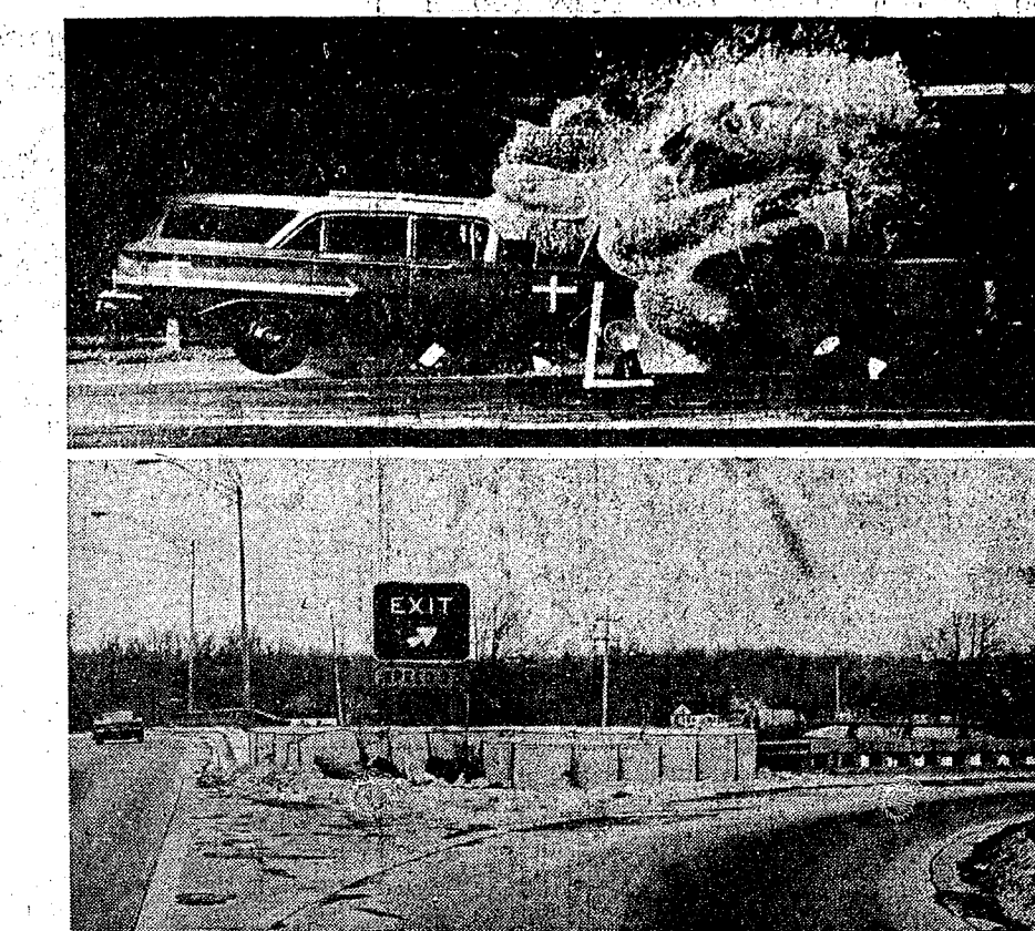
DOING THE JOB: Clusters of plastic barrels, partially filled with sand, are proving effective in preventing serious accidents at several exits on Michigan freeways. Top photo shows vehicle crash into barrels at high speed. Below is aftermath of collision at I-496 Freeway exit in Lansing. In seven accidents at this site, drivers have been able to back off and continue on.
